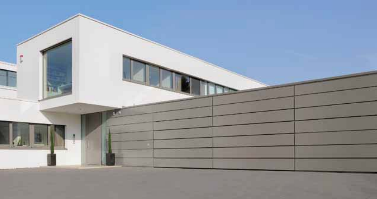
On-site cladding with aluminium compound board
